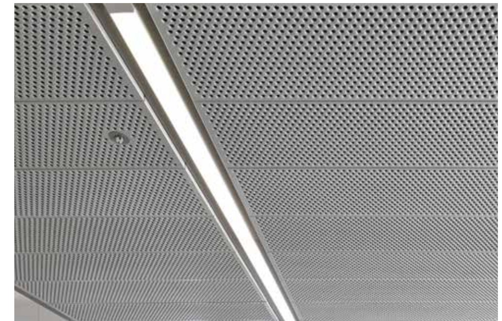
Recessed linear light fittings within unique raft system
