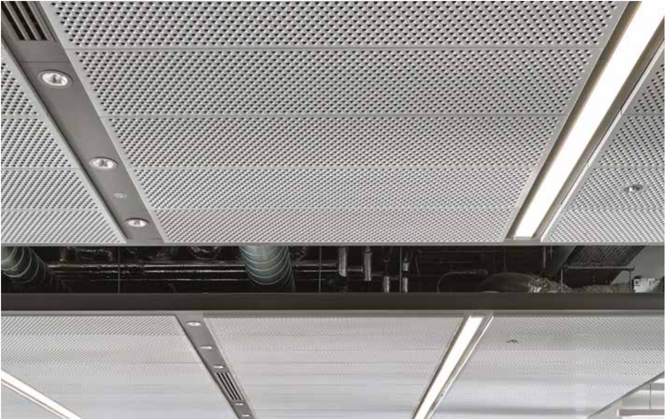
New four pipe fan coil air-conditioning in a unique raft system
