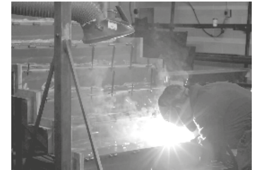
Chay Wheeler on site welding the suspended stair
