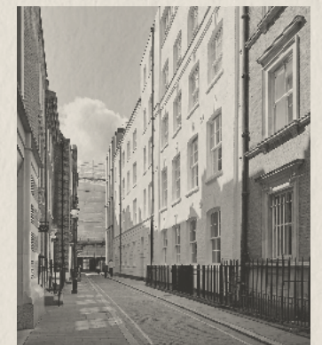
The retained buildings in Took's Court
