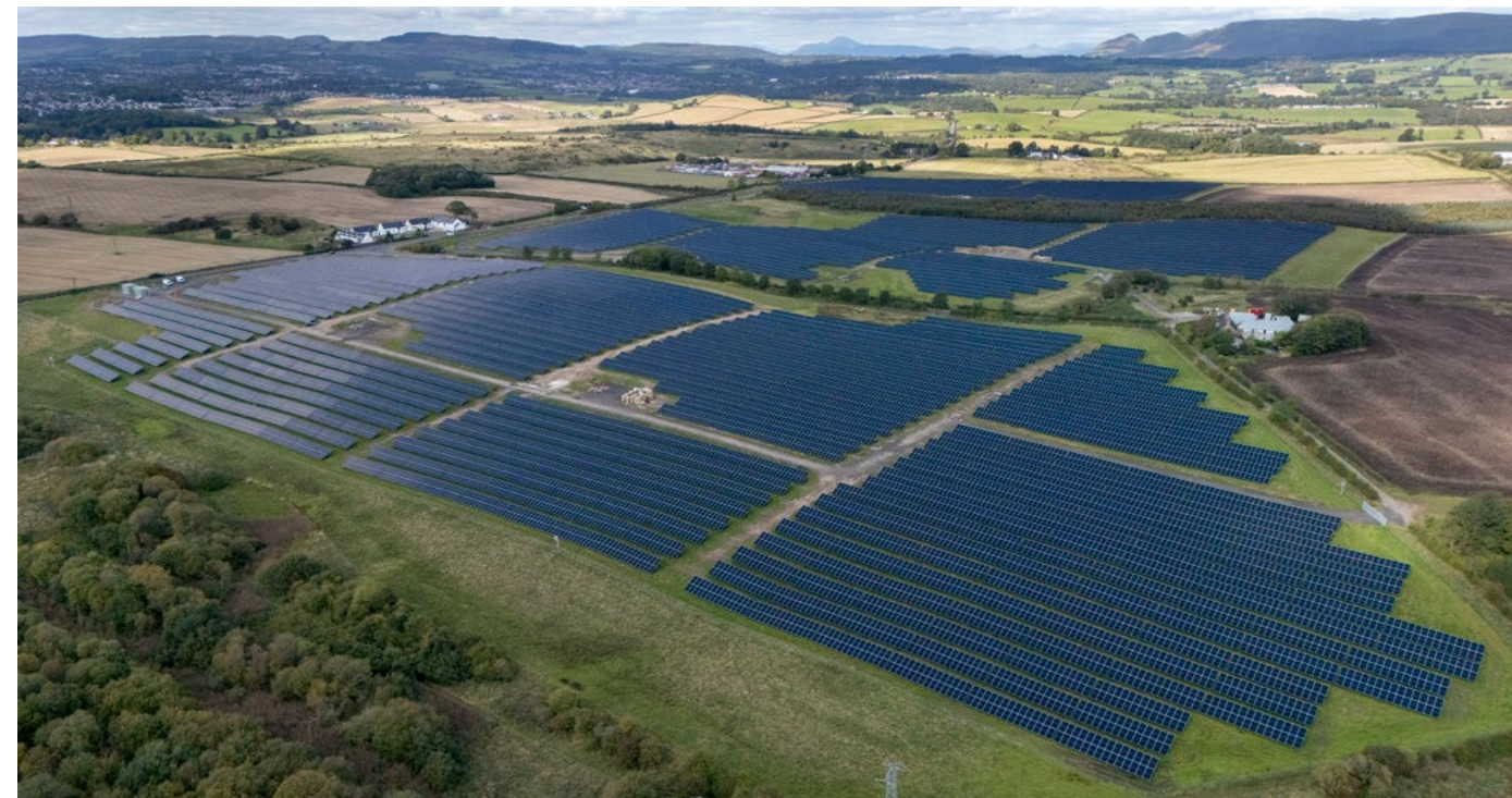
Lochfauld Solar Park
