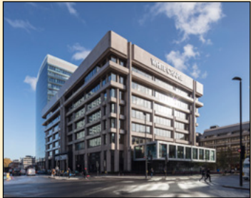
THE WHITE CHAPEL BUILDING
