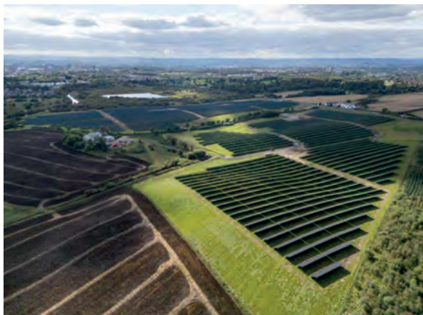
Lochfauld solar park – Scotland
