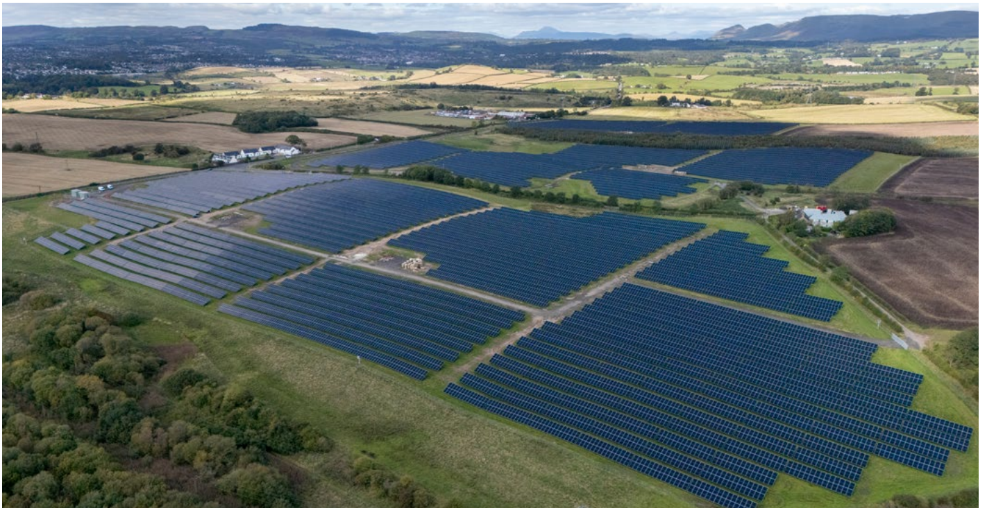
Lochfauld Solar Park
