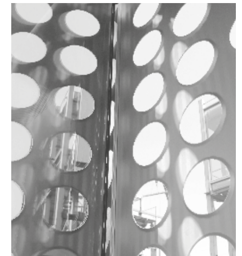
Screens punched with Prouvé-inspired portholes reduce solar load and protect from wind
