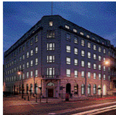
21 Grosvenor Place, Belgravia, SW1 Office refurbishment Architect: Squire & Partners
