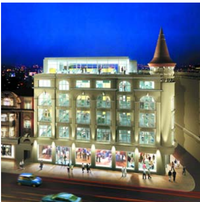
135-155 Charing Cross Road, WC2 Office/retail refurbishment Architect: John McAslan & Partners
