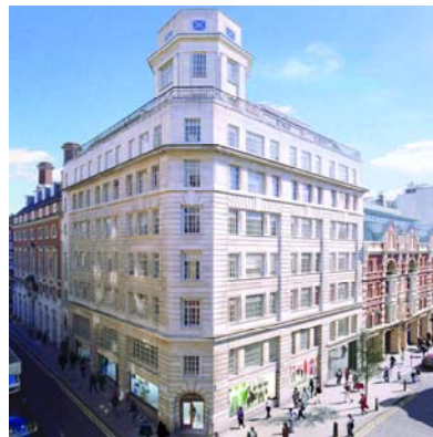
Tower House, Covent Garden, WC2 Office/retail refurbishment and development Architect: Lifschutz Davidson
