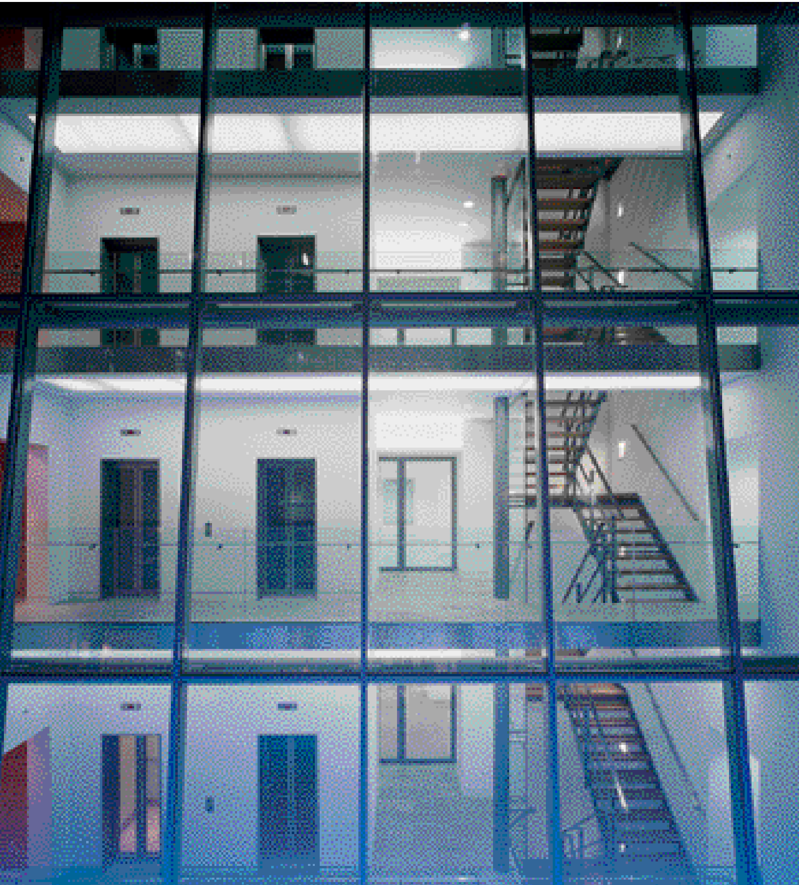
Panton House, rear glazed façade
